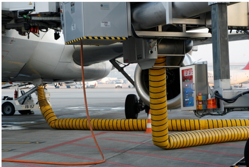
Figure 9 Hose for pre-conditioned air at pier A.
