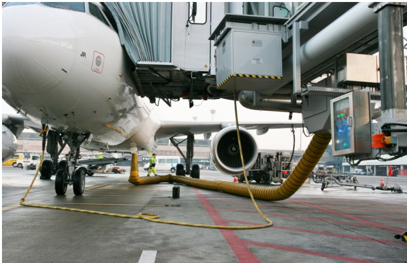
Figure 10 Hose for pre-conditioned air at pier B.
